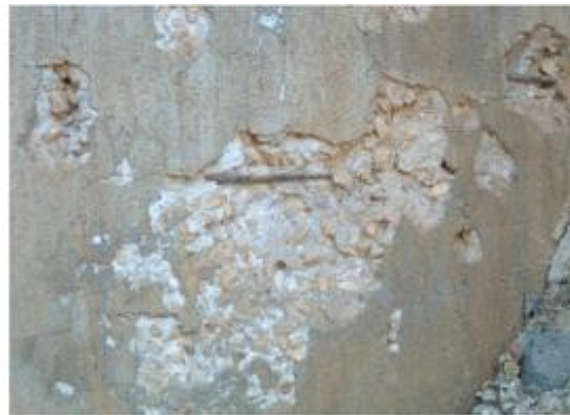
Fig. 30 concrete spalling at massive abutments
