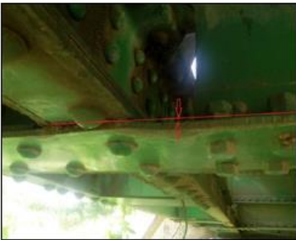
Fig. 24 Out of plane deformation at the bottom plates of the truss-girder connection
