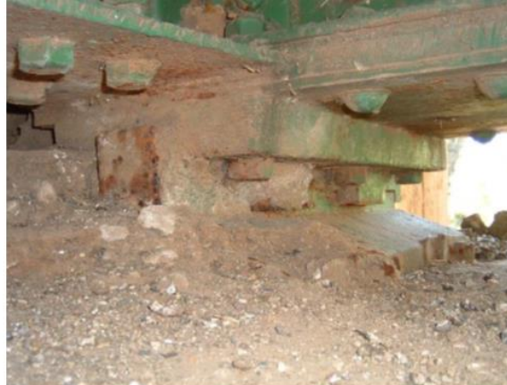
Fig. 34 Corrosion damage at fixed bearing
