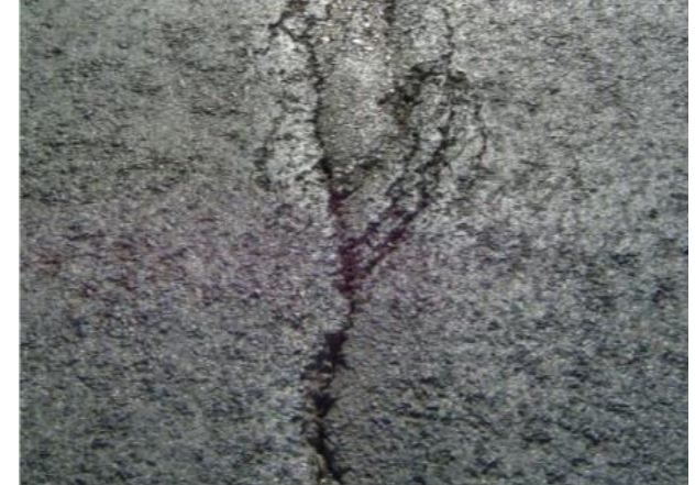
Fig. 37 Asphalt defects near and over joints
