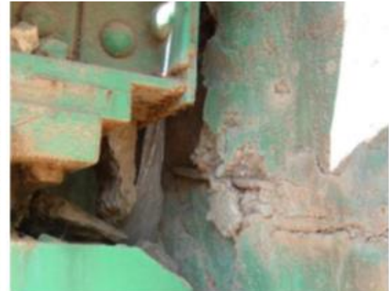
Fig. 32 damage to closing wall near supports at massive abutment
