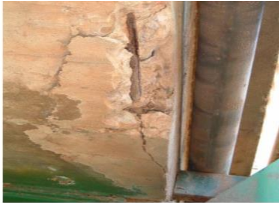
Fig. 27 Spalling and delaminations along the deck slab edge (typical along the edges)
