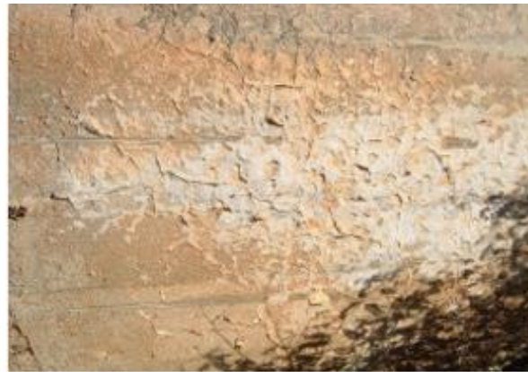
Fig. 31 Concrete surface abrasion at massive abutments
