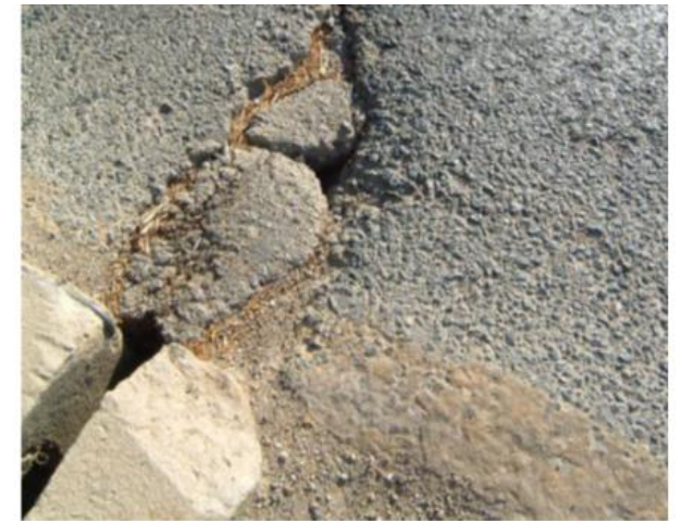
Fig. 38 Asphalt defects near and over joints
