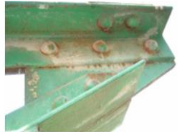
Fig. 26 Corrosion of truss member (typical condition) Corrosion between riveted angels and plates
