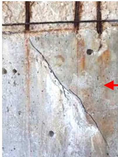
Hairline shear cracks
