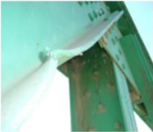
Fig. 21 Local collision damage to members few locations
