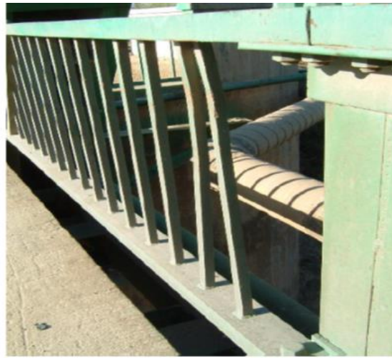
Fig. 36 Safety barrier collision damage
