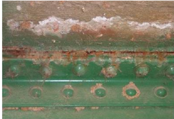
Fig. 28 Corrosion at the connection between transverse girder and the deck slab with efflorescence due to water penetrating in between the girder upper
