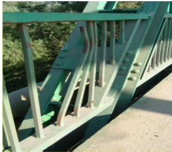
Fig. 35 safety barrier collision damage
