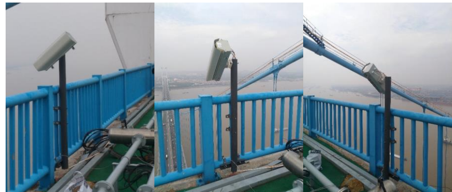
Cameras installed at top of pylon
