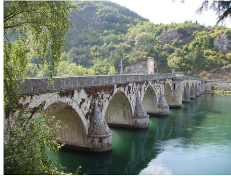
Fig. 4. Vegetation growth -the bridge is at risk from self-sown vegetation
