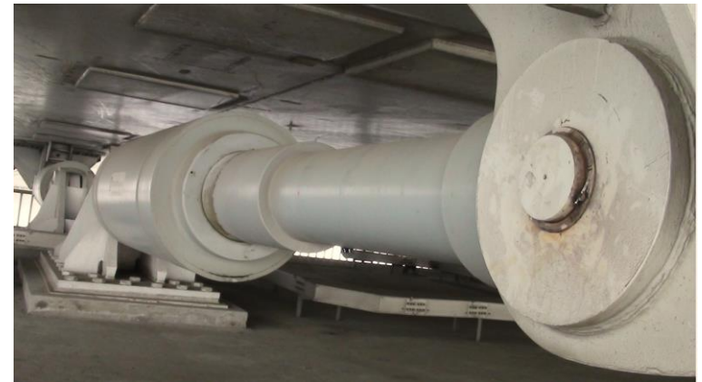
67DP-17621-01 dampers of Taylor company Applied at Sutong Bridge
