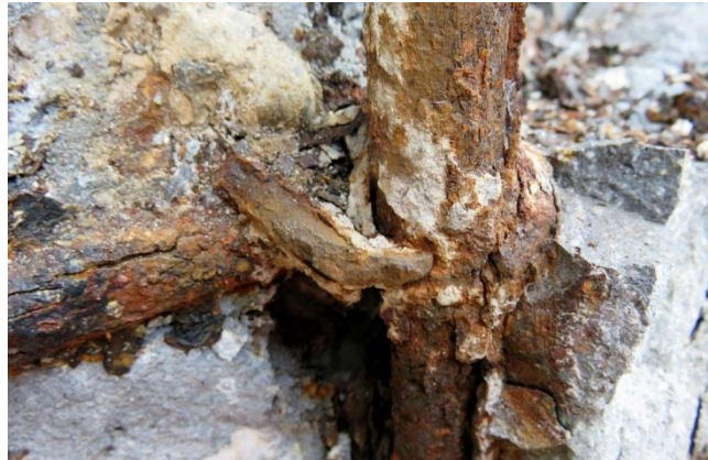
Fig. 2: Fully corroded cross tie in hollow box bridge column with improperly or sub standardly positioned transverse reinforcement placed on the inside of the longitudinal bars
